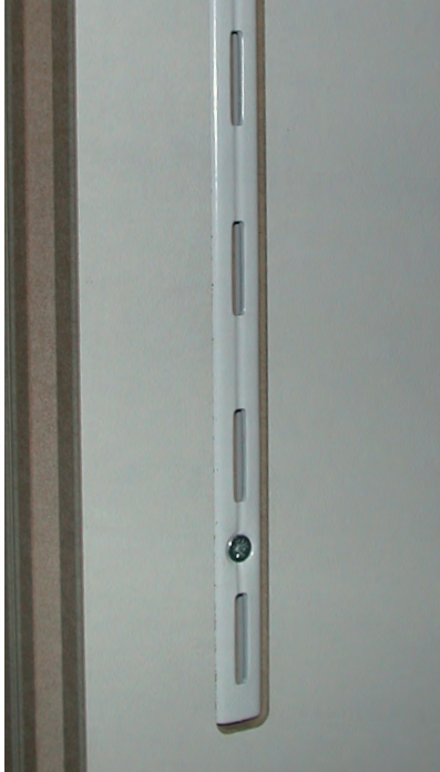
Schlitzschiene, eingenetet Slotted rail set in groove
