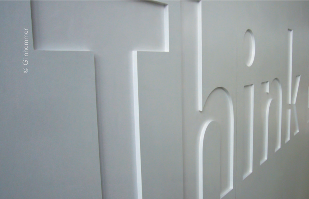
Schrift in G40 CLASSIC Leichtbauwand gefräst. Font milled in G40 CLASSIC lightweight wall.
