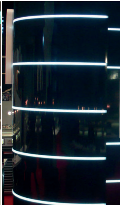
LEDs in Wandfläche eingearbeitet LEDs installed into wall surface
